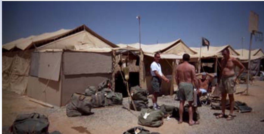
TABUK, Saudi Arabia – Members of the 142d Airlift Squadron build a tent city in the middle of the Saudi desert, March-2003. The base, which became the hub of airlift operations during OPERATION IRAQI FREEDOM, was devoid of housing, infrastructure and facilities when these Airman arrived. (Courtesy photo)
