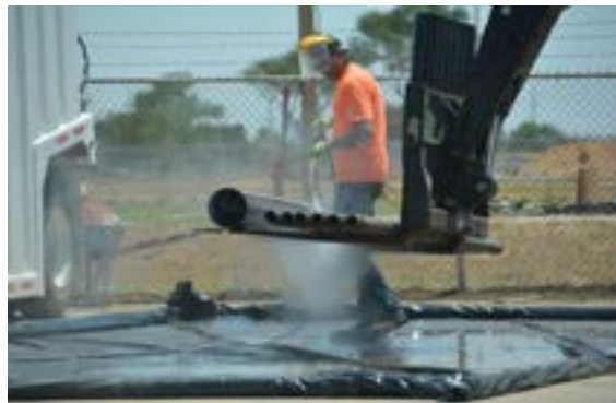
An Air Force contractor prepares drilling rig equipment at the former Reese Air Force Base near Lubbock, Texas, June 28, 2020. The Air Force Civil Engineer Center is moving forward with environmental remediation and will install twenty-five monitoring wells in a 12 square mile, down gradient area from the former base, to further determine human and ecological health risks, source areas, and migration patterns of Per-and polyfluoroalkyl substances (PFAS) contamination there. (U.S. Air Force photo by Sriram Madabhushi).
